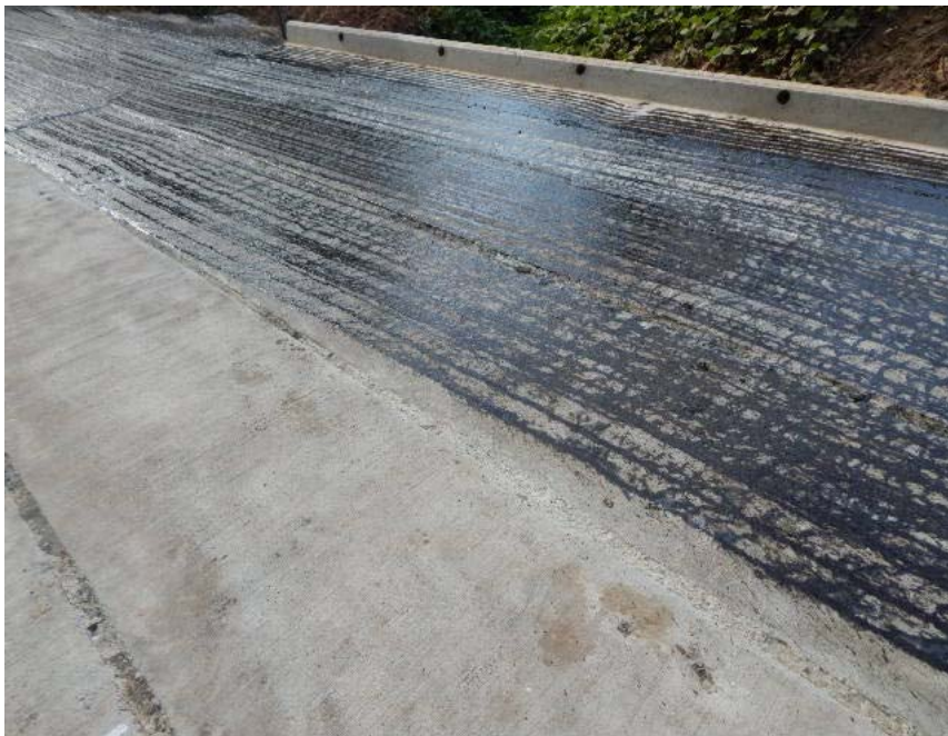
VIEW ACROSS TOP OF DECK
